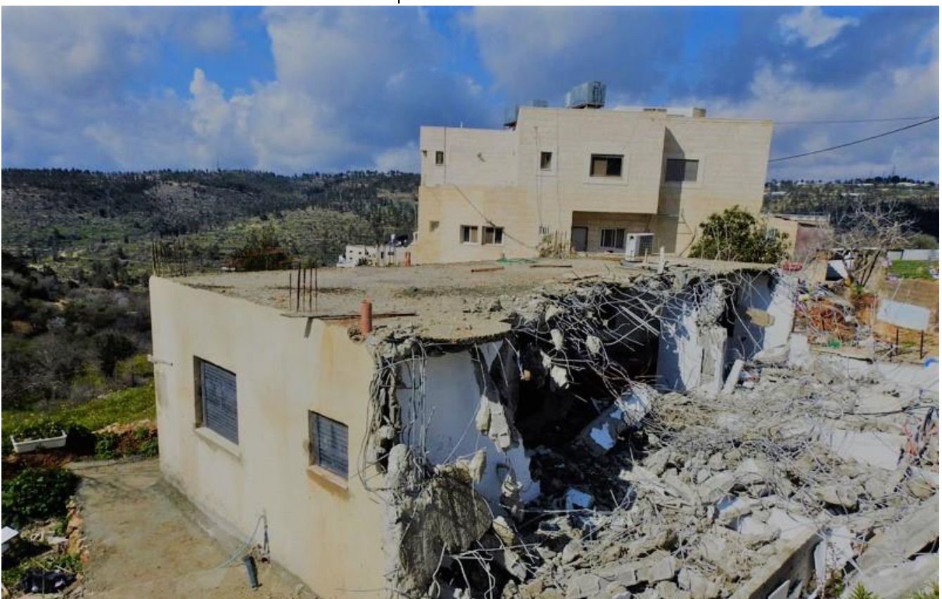
Abu Al-Haija family demolished house, November 2020, LRC®
