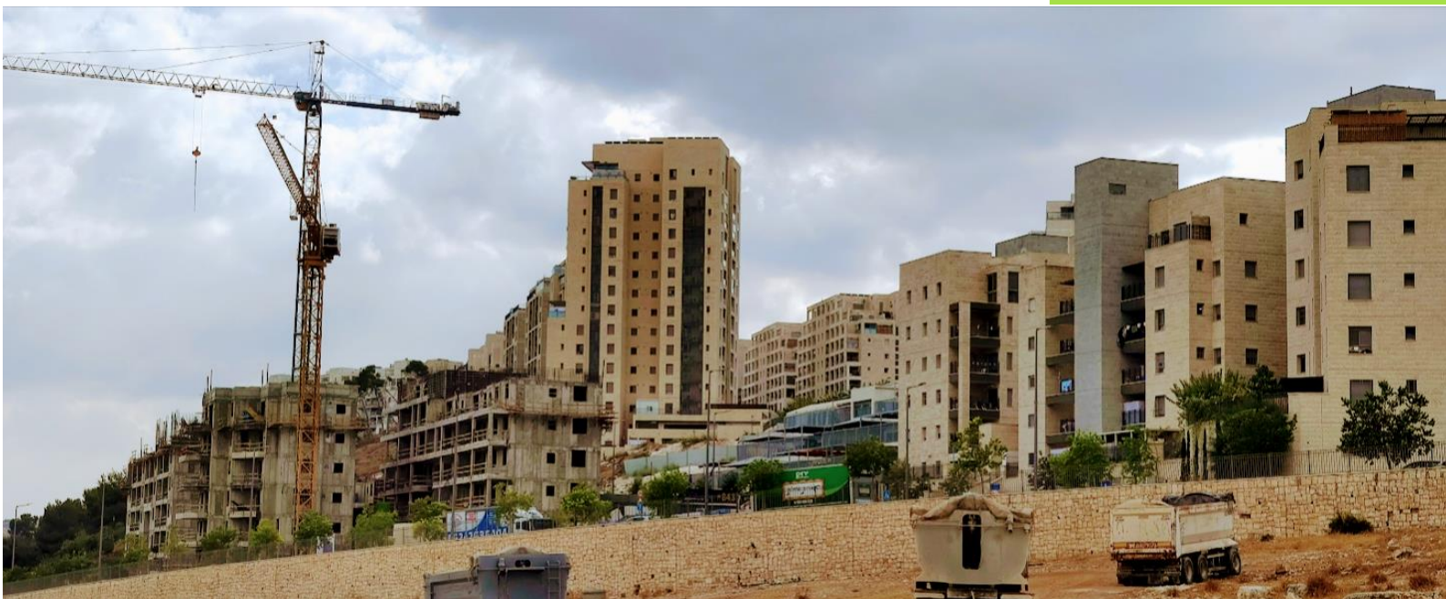
New buildings in Har Homa
