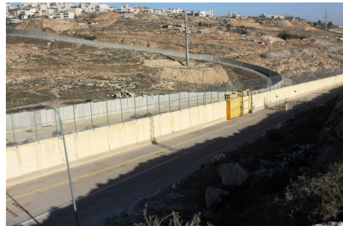
Part of Route 4370, which is divided in the middle by an eight-meter high wall
